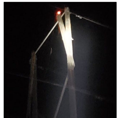
Burnt crossarm on transmission structure (below)
